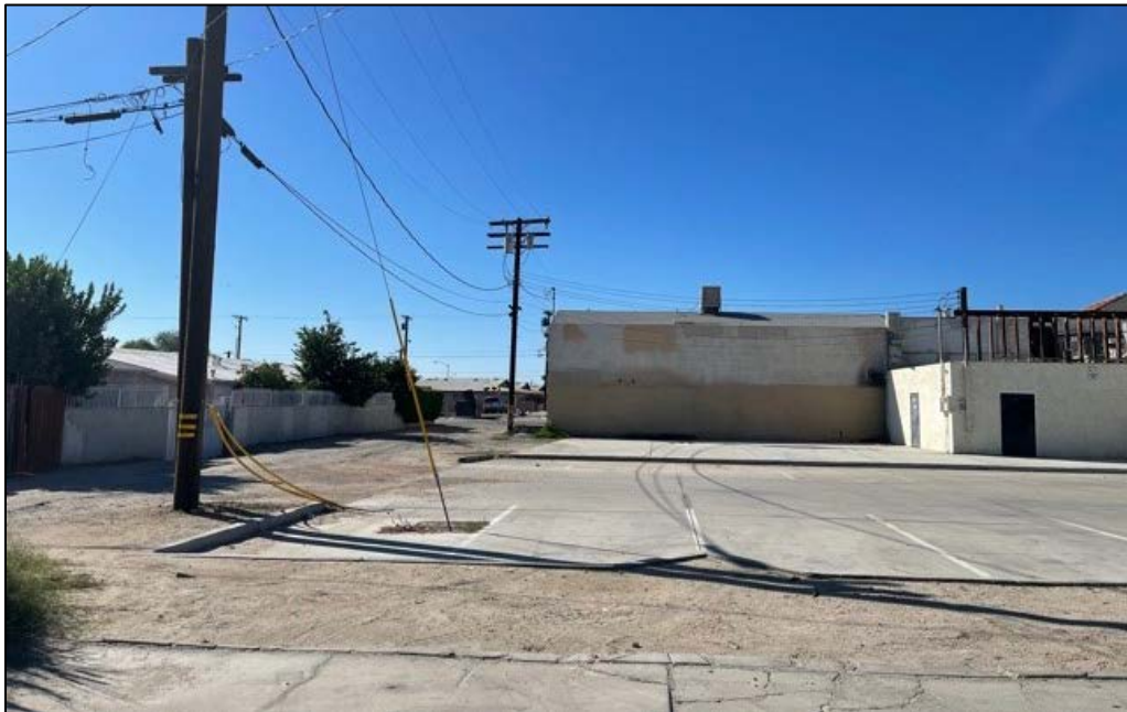
Rear of Property and Parking Area
